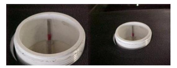
3) Check water levels frequently after every use to ensure optimal performance of a/c unit.
